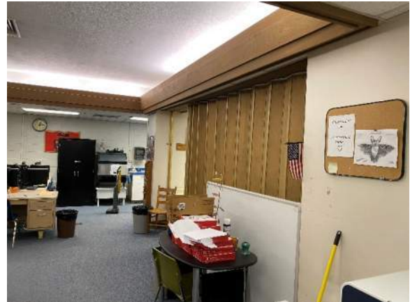
Fig. 15: Windowless space at core of upper floor
