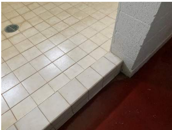
Fig. 20: Curb at shower room
