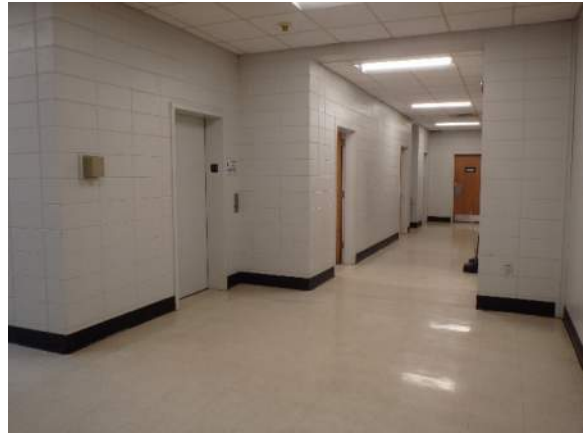
Fig. 16: Upper level dead end corridor
