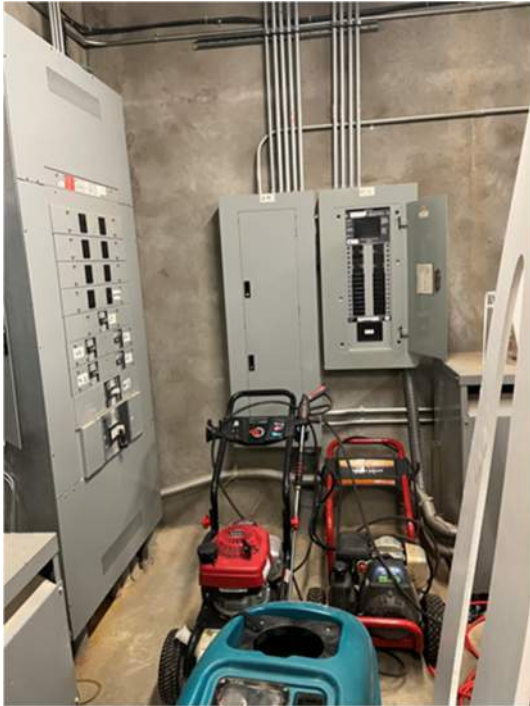
Fig. 9: Existing access to panels
