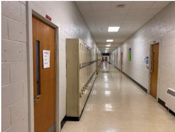
Fig. 4: Narrow corridors with 4" CMU walls
