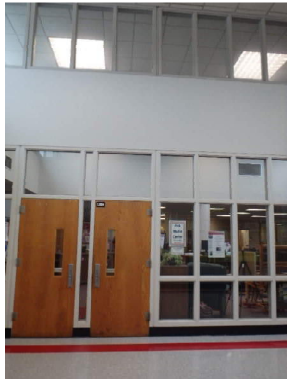
Fig. 5: Wire glass at lobby windows.
