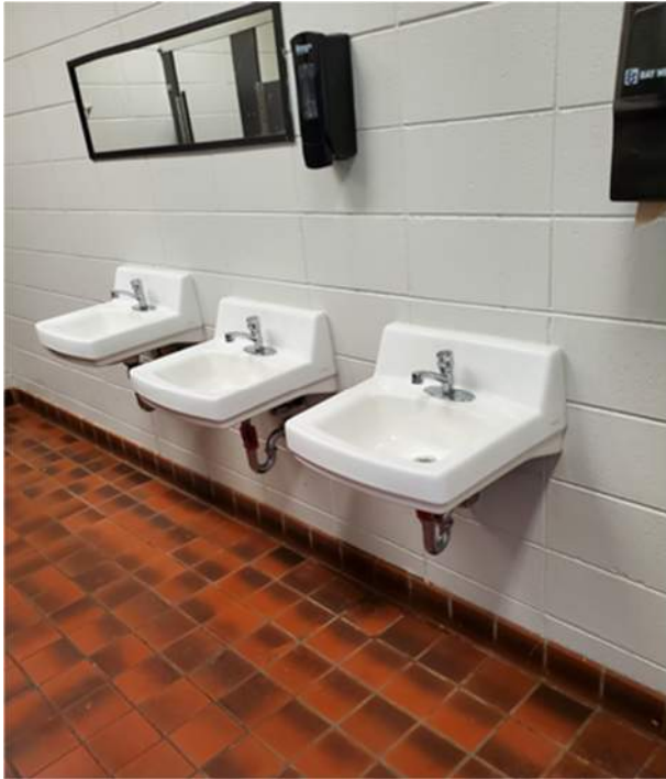
Fig. 6: Group restrooms, plumbing fixtures.
