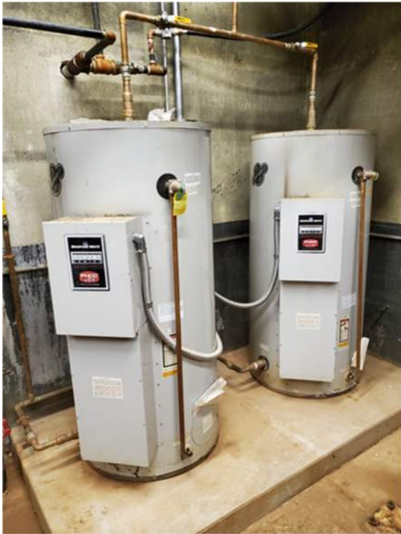
Fig. 11: Water heaters
