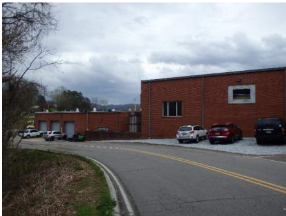
Fig. 2: Impromptu parking beside Vocational Building
