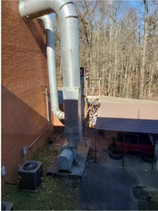
Fig. 10: Dust collection system
