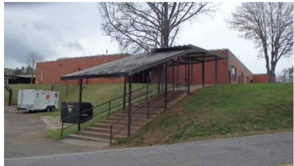
Fig. 4: Covered walk outside security fencing beside Media Center
