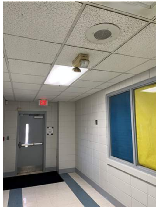
Fig. 12: Existing emergency light fixture
