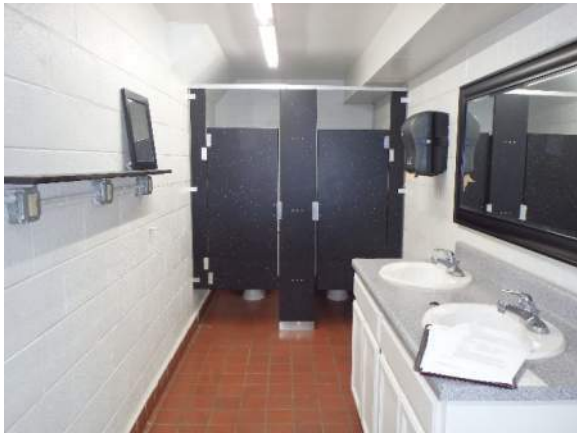
Fig. 19: Non-accessible bathrooms in locker room.
