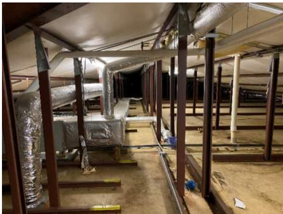
Fig. 1: Overbuild roof system, Main Building
