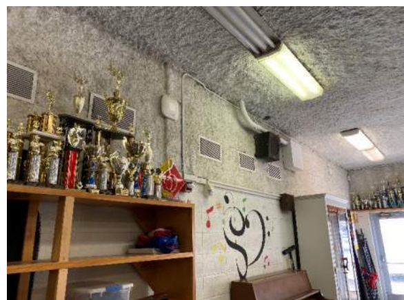
Fig. 6: Spray-on retrofit acoustical insulation
