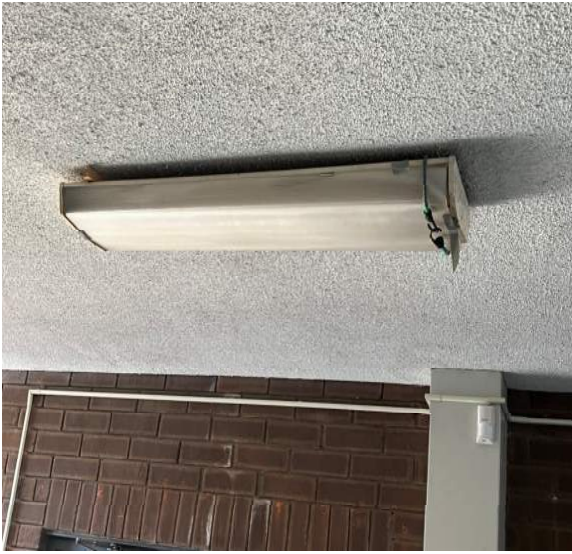
Fig. 15: Existing lobby light
