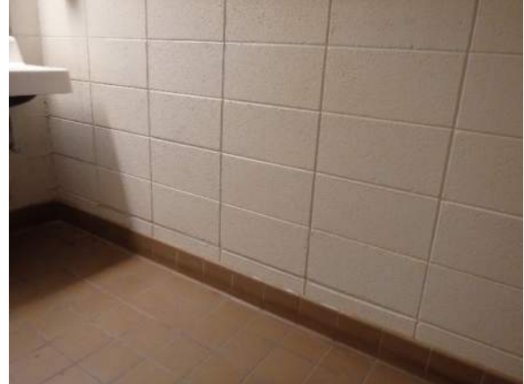
Fig. 3: Subsidence at upper level slab
