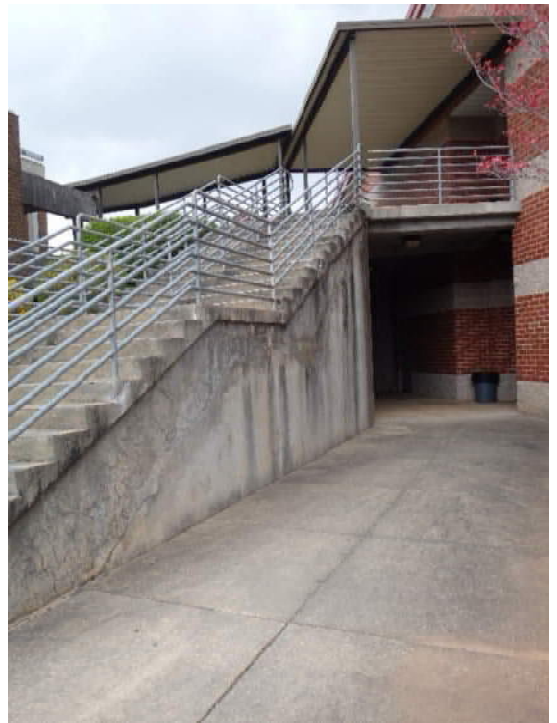
Fig. 8: Deteriorated stairs.
